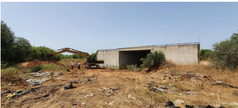
Area cleaning of Varda I/C ανδ top soil removal (k.p.: 33+000)
