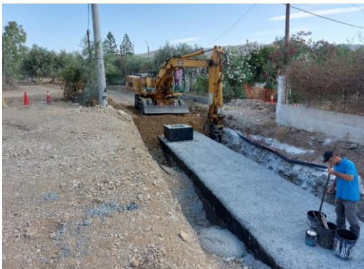
Construction of open ditch to the side road of the Motorway
