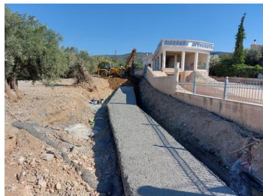
Construction of the side road embankment
