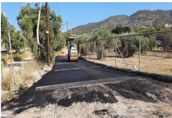
Asphalt Works of the local streets of the Motorway
