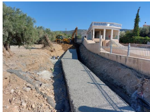
Construction of the side road embankment
