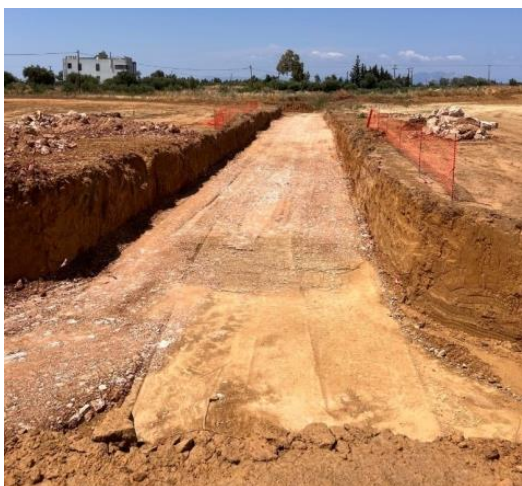
Excavation of box culvert L609A, L609B (k.p.: 17+560,44)
