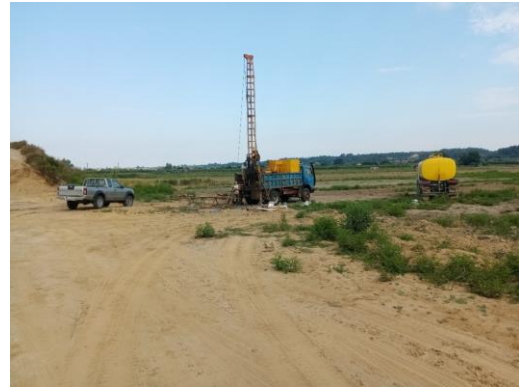
Exploratory/Sampling boreholes from k.p.: 73+000 to k.p.: 73+500
