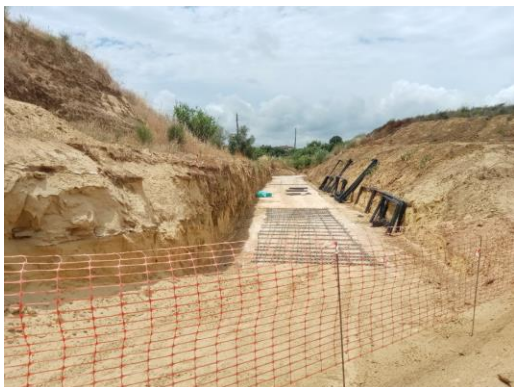
Construction Works for sewer L402
