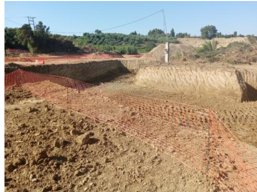
Construction Works for Underpass K848
