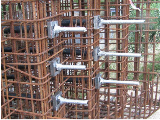
Placement of Freyssibar Prestressing System in the pile caps
