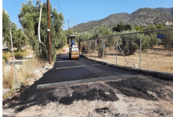
Asphalt Works of the local streets of the Motorway
