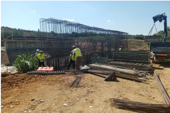
Construction Works for Sohias bridge B881 (piers)
