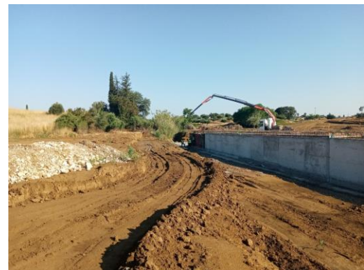
Construction Works for sewer L406
