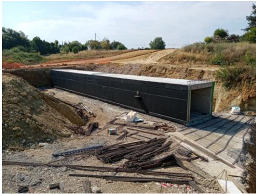
Construction Works for sewer L428
